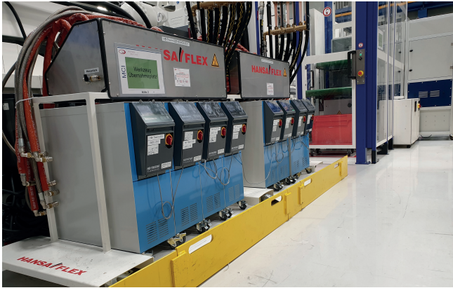
Fig. 1. Up to ten Thermo-5 temperature-control units per machine are clearly and neatly arranged © HB-Therm
